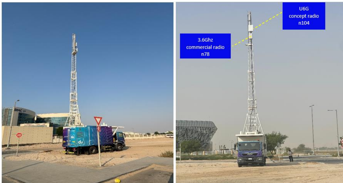
Figure 2. Suburban COW site with upper 6 GHz and 3.6 GHz radios
