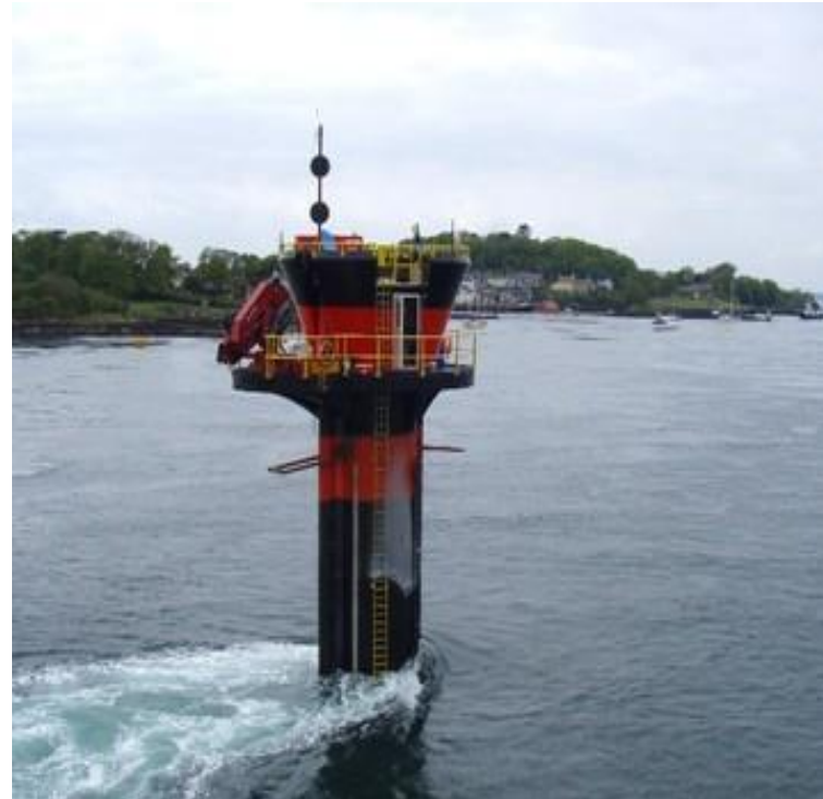
First grid connected tidal stream generator, Ireland.
