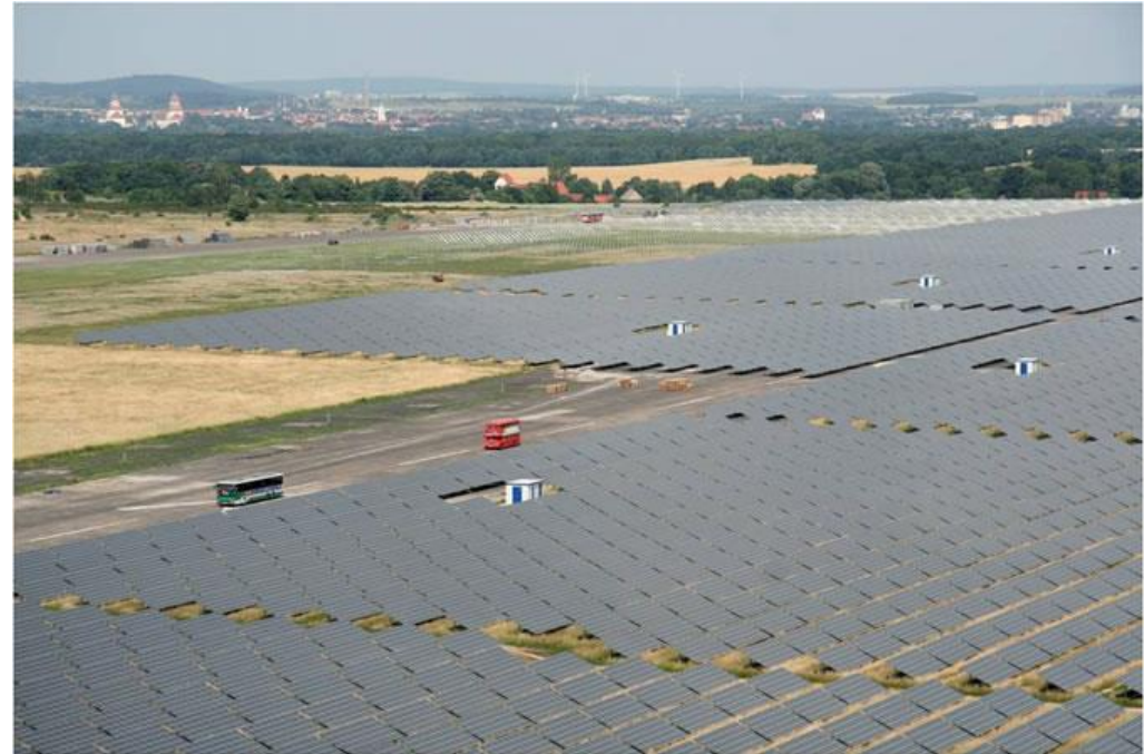
Waldpolenz Solar Park, Germany
