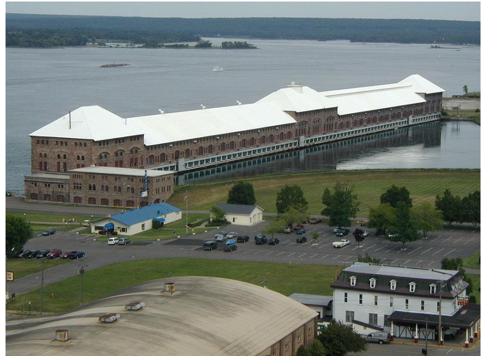
Saint Marys Falls – run-of-the-river plant, .
